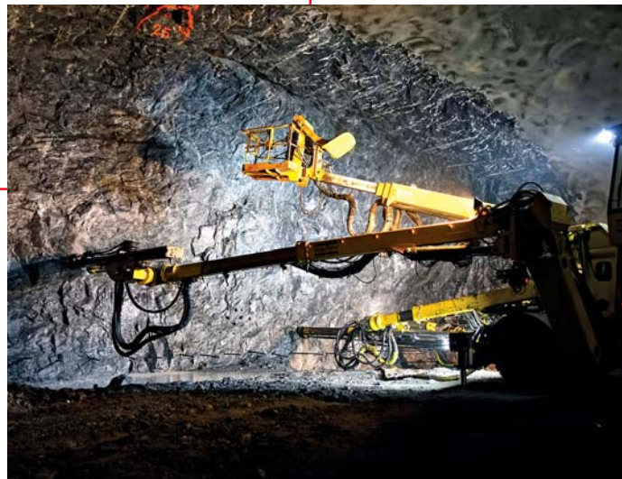
Výstavba tunelu Skarholmen, Stockholm Bypass, Stockholm, Švédsko Construction of Skarholmen tunnel, Stockholm Bypass, Stockholm, Sweden
